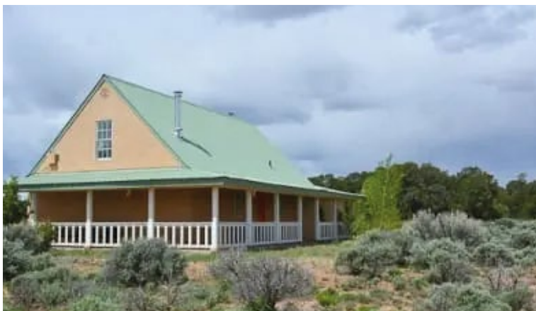
Off-grid, passive solar adobe home for sale in Tres Piedras, N.M. GREENHOMESFORSALE.COM
