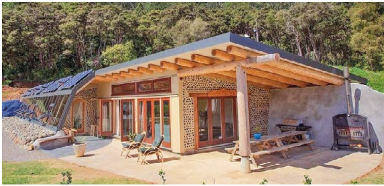
Custom Earthship: Off-grid sustainable/regenerative building via thermal dynamics and passive solar made of natural and upcycled materials. Earthships can be completely off-grid or partially off-grid. PANGEABIOTECHTURE.COM
